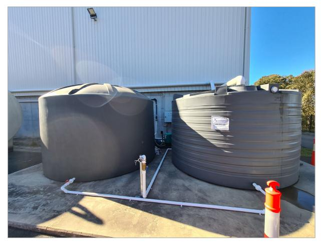
Photograph 4: Existing static water supply
